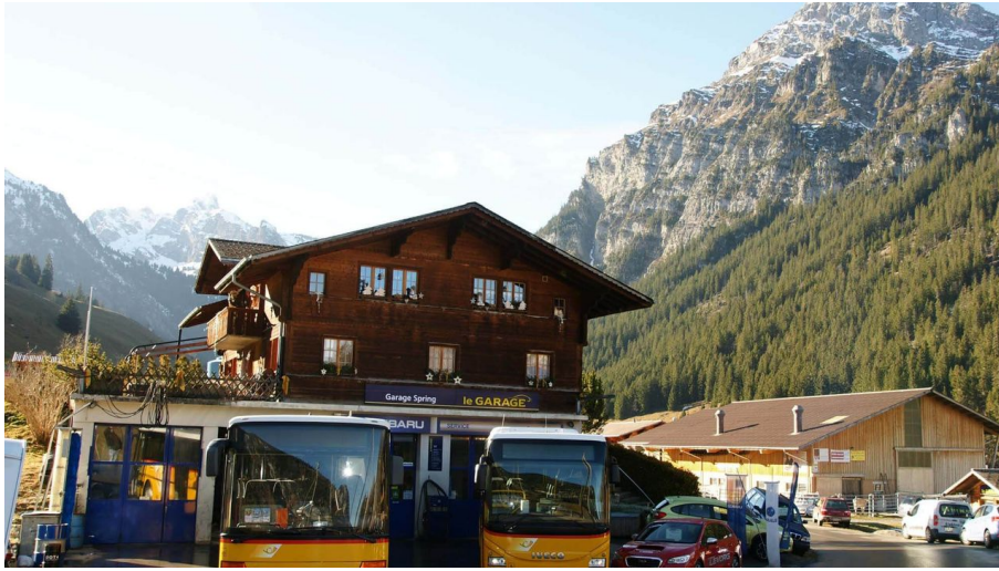
Garage Spring Schwenden - © Spring AG Schwenden
